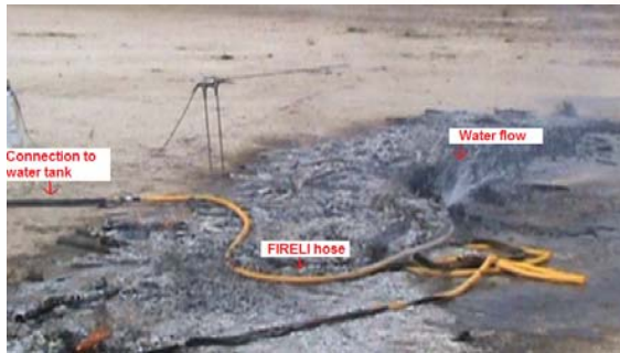
The FIRELI hose during the smoldering-glowing phases of the fire
